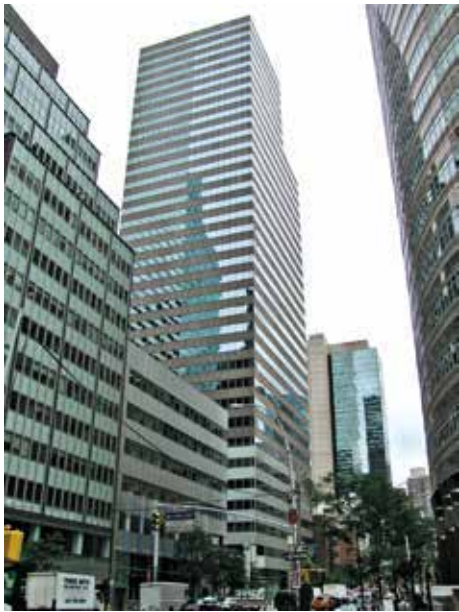
Bangunan pejabat Third Avenue, iaitu lokasi Pejabat Perwakilan di New York The Third Avenue office building in which the Bank's New York Representative Office is located
